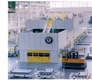
Production line Automatisation and transport kinematics
